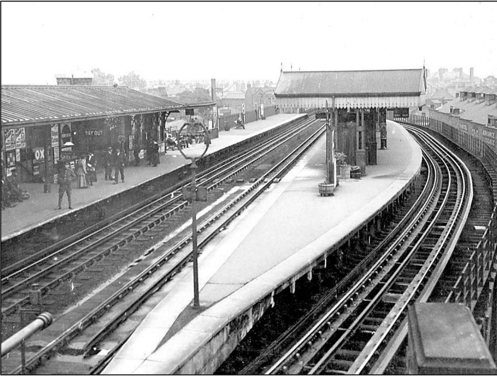
**Left:** Insofar as Putney Bridge was concerned, the Down platform was converted into a bay platform and a new third platform was added 'around the back' through widening. The third track became operational from 24 April 1910 with the completion of the project two months later. This view looks east from the westbound (Down) side. From 12 January 1911 the buffer stop in the new bay platform was replaced by oil resistance buffer, its outer end just visible at lower left.
