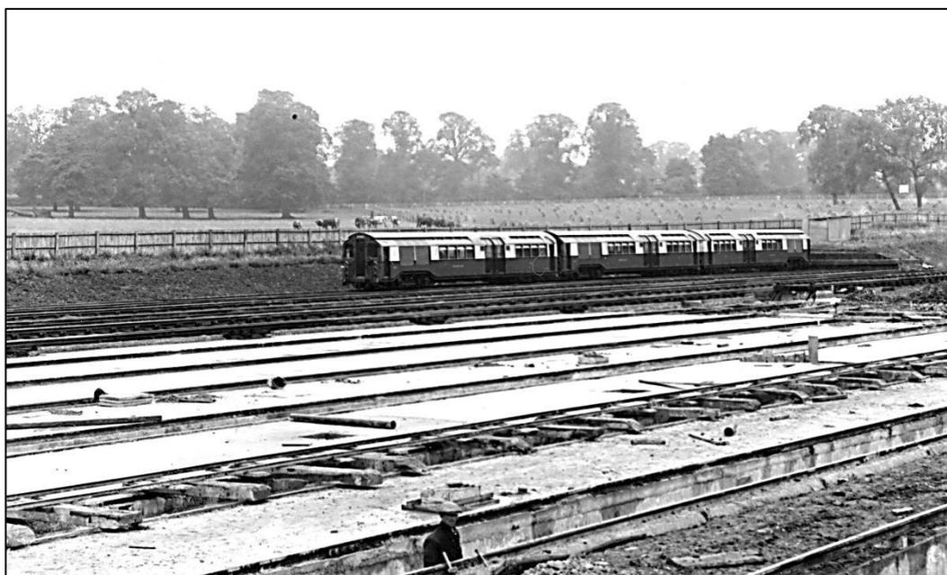
*Figure 1: Morden depot about mid-1925, showing three 1924 Met. Carriage motor cars stored on No.1 road after delivery. The depot is a long way from complete. They have dug the pits and concreted some of them but they haven't put up any of the building structure yet. Storing cars for long periods leads to quite rapid deterioration and I suspect some cars needed work before they were fit for service. Photo: B.R. Hardy collection.*
