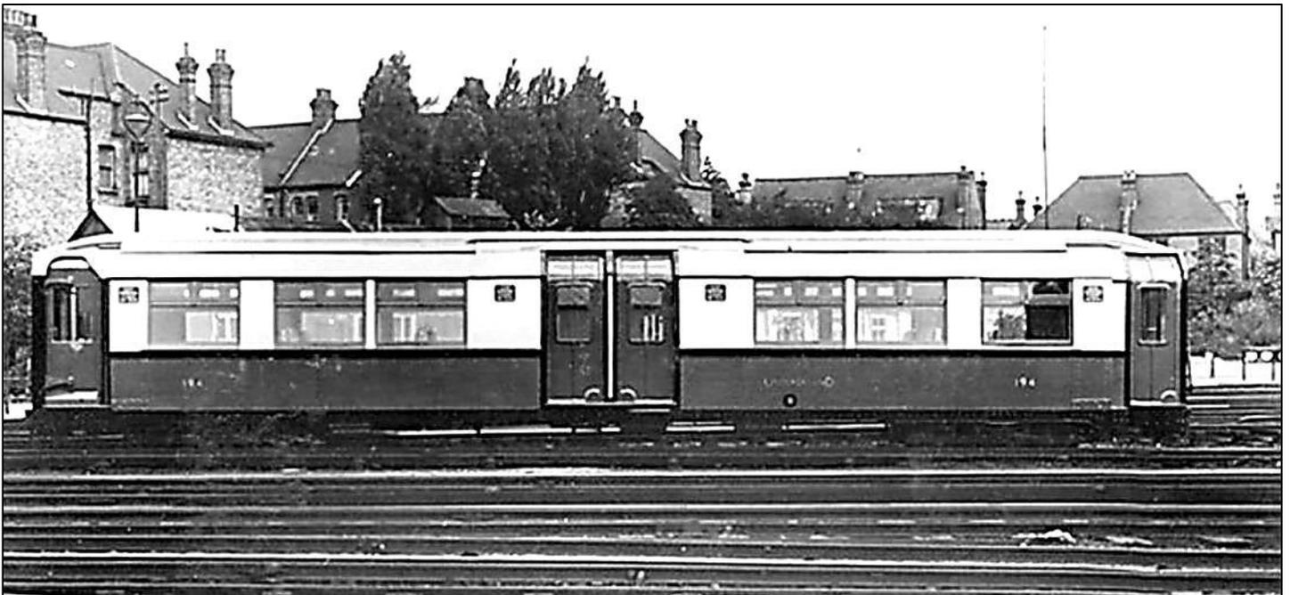
*Figure 2: Hampstead gate stock trailer car No. 194 in the yard at Ealing Common depot after its conversion to air door operation. The two end platforms have been enclosed and side doors provided while a double doorway has been cut in the centre of the car. The layout was similar to the 1920 Cammell Laird stock. The door on the west end of the car is a special design to test the concept of a rotating door rather than a sliding door. Photo: LT Museum.*
