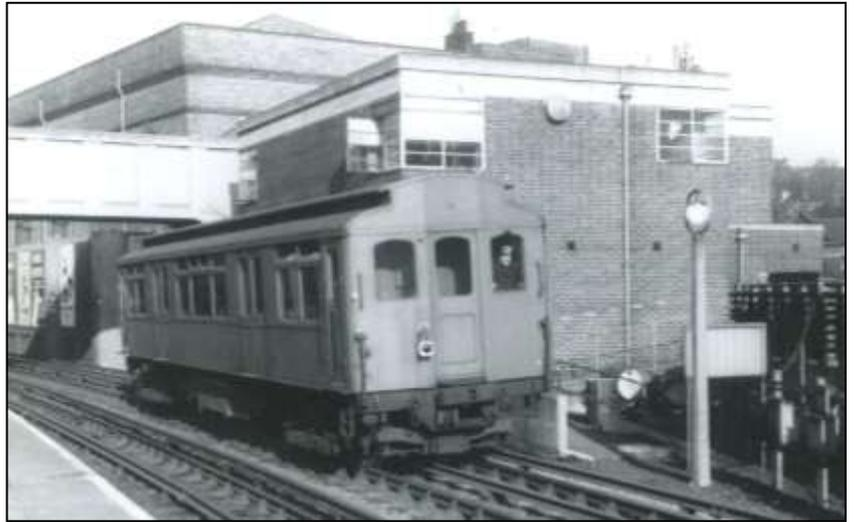
*Fig 3: “Acton Shuttle” car 4176 (G23 Stock) departing Acton Town for South Acton with the former trailing end leading. Only a single headlight and tail light was provided at this end for the conversion work carried out in 1940. Immediately behind the car is the Acton Town signal cabin and behind that is the substation. The service was withdrawn on 28 February 1959 and this car and its sister, No.4167, were officially scrapped on 25 May 1959.*
