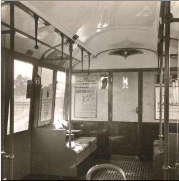
*Fig. 3: Interior of O Stock "D" motor car with end ventilation grille which was unique to this stock.*
