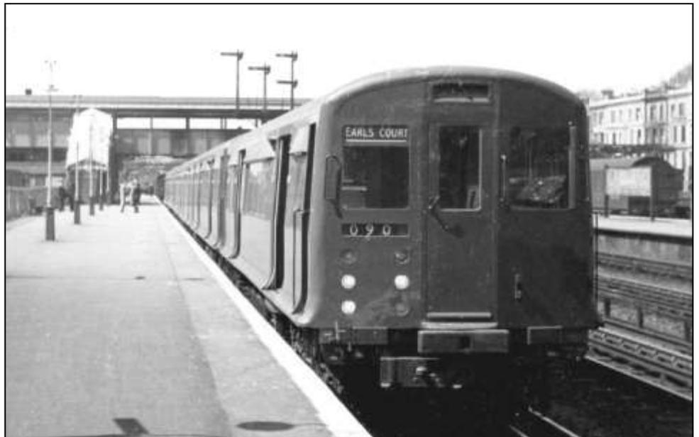
*Fig. 3: New 6-car R Stock train at Olympia in the early 1950s. This is one of the early deliveries. The driving car still has non-stop indicators either side of the second set of double doors and passenger door open buttons are in place. The cab front shows the destination blind over the offside cab window and the individually switched marker lights below the train set number. Just to the right of the train set number is the flag*
