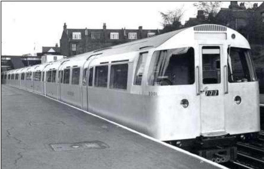
*Figure 1: The first 4-car unit of 1967 Tube Stock (Unit No. 3001) on test at South Ealing, 3 November 1967. As a driver on the Piccadilly Line at the time, I used to see this unit regularly. It was sometimes stabled in Northfields depot where I was based, so I would sneak a look inside from time to time. There was a lot of instrumentation, I recall. The testing was done on the fast tracks while the Piccadilly Line service used the local tracks. LT Museum photo.*
