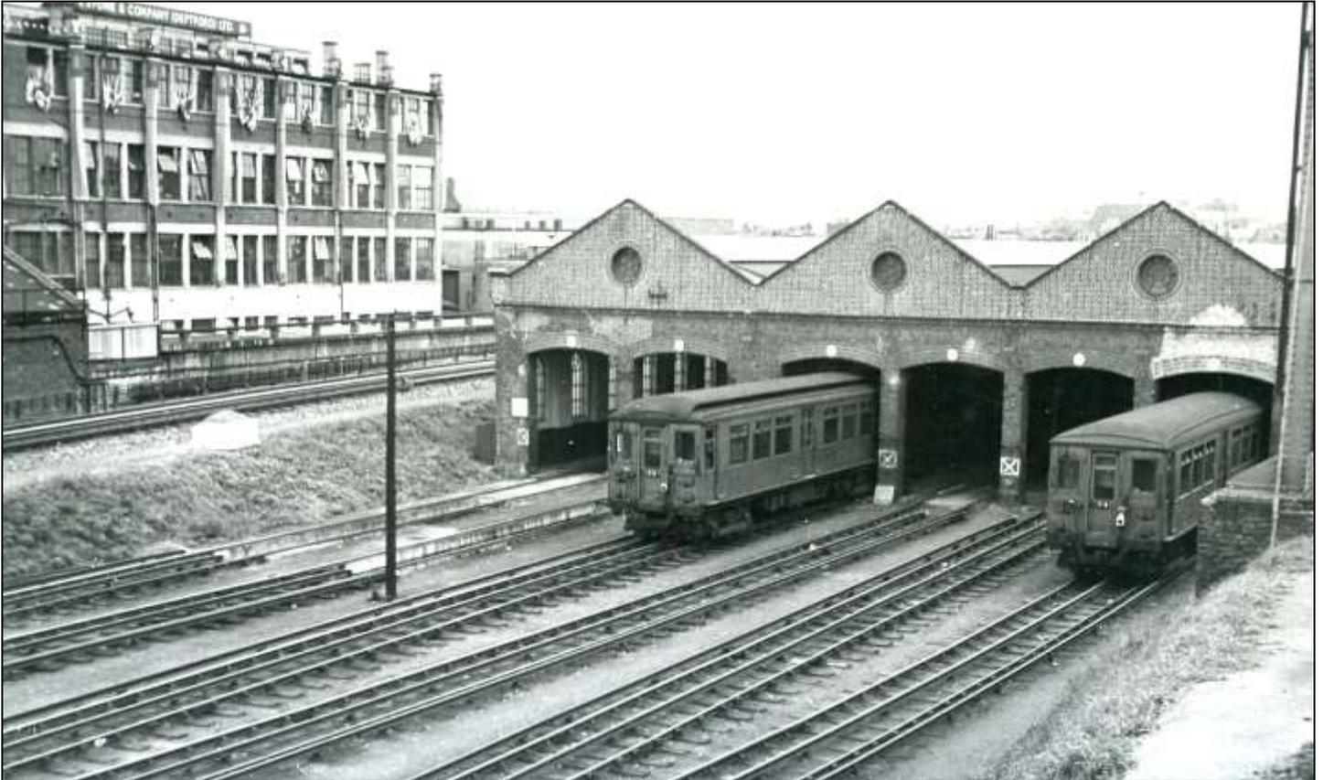
A trip to New Cross depot in the early 1950s (*above*) saw two trains of H Stock stabled – a 1910/11 C or D Stock motor on the left and a 1914 E Stock motor car on the right. F Stock took over on the East London Line in 1953 and some ten years later Q Stock replaced the F Stock.
