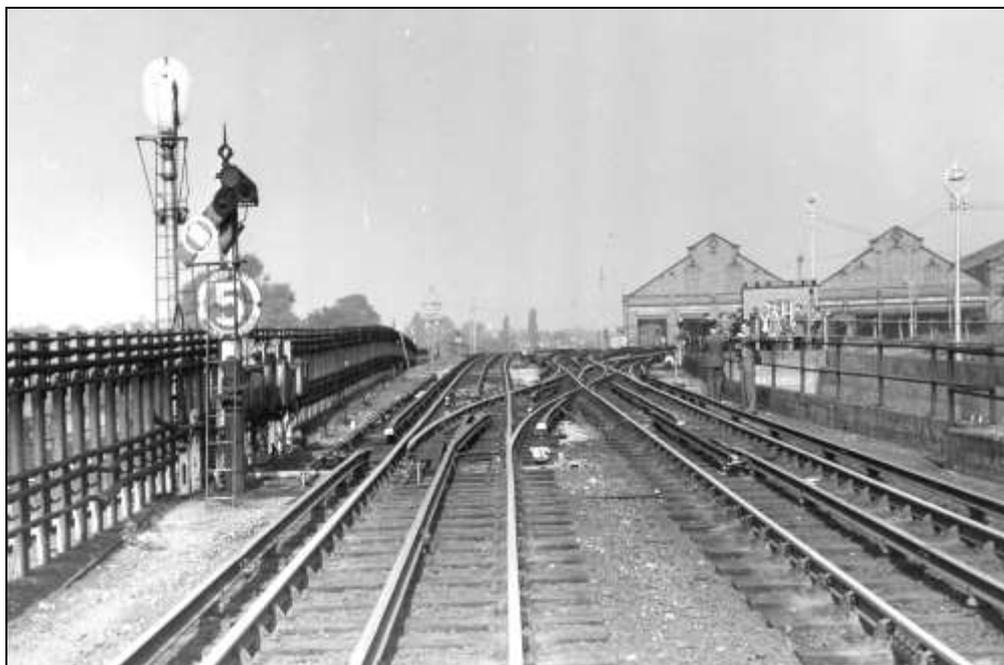
This picture was published in *Underground News* back in 1999 and shows the signal that was nearly always in the 'off position' – it was used by District trains stabling in Ealing Common depot direct from Acton Town station onto 16-20 roads on the left. The signal was only put to danger if a train was required to be worked to the roads to the right, i.e., 1-15. It was abolished when direct access to the depot from Acton Town westbound was abolished in 1965.
