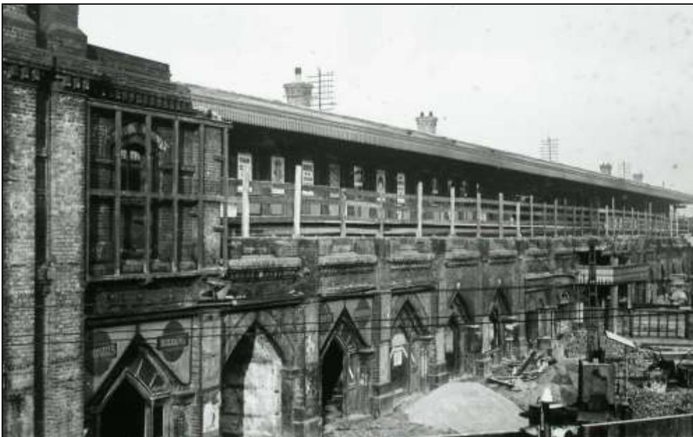
Work has now begun at Finsbury Park to make room for the overhead structure for the future Northern Line tracks and island platform station. The station frontage is in the process of being demolished and even though a small section of the canopy remains (on the right), the whole area is now a working site.
