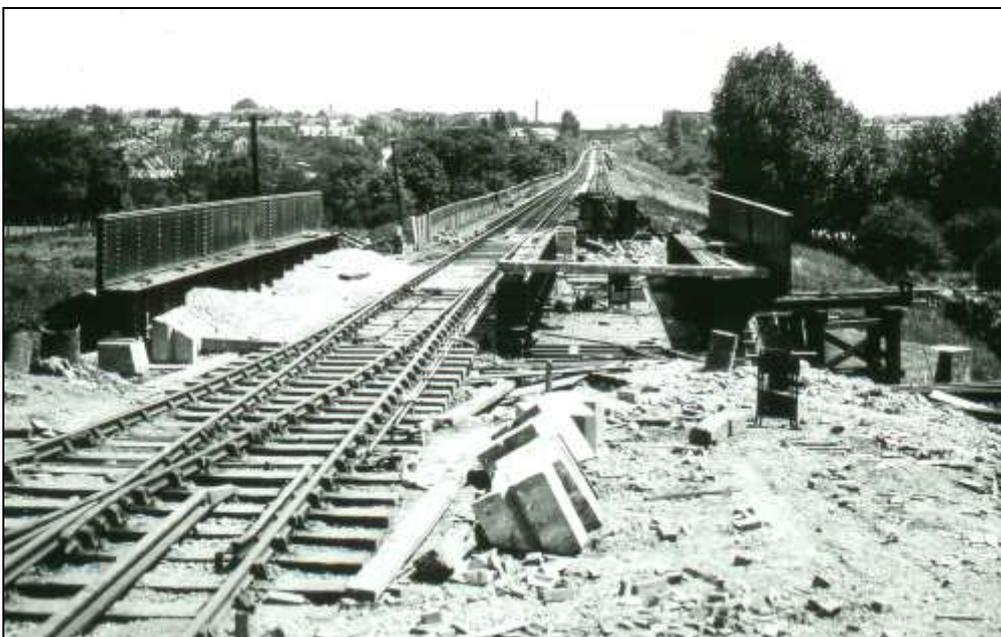
Looking south between Mill Hill East and Finchley Central on the Edgware branch with work progressing on bridge reconstruction in the foreground to provide the second (northbound) track. Sections of current rail have already been laid on the southbound line on the left.
