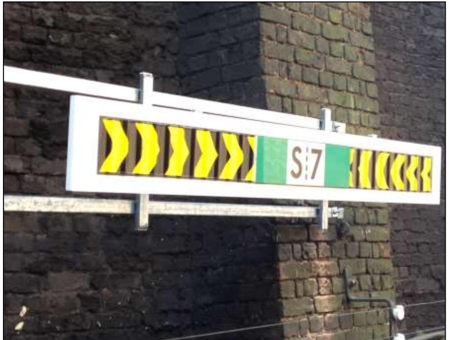
They have a ribbed front edge which catches the trains headlights, very useful when they are placed in a dark tunnel! The view (*Below*) at the east end of East Ham shows the ‘ribbed’ edge.
