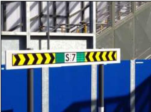
**NF 51/12** – New S7 stopping markers have been put up at Bayswater (*Right*), about one C Stock car’s length beyond the platforms. They are of a different design to the other S8, S7, SS boards around (*Above*).
