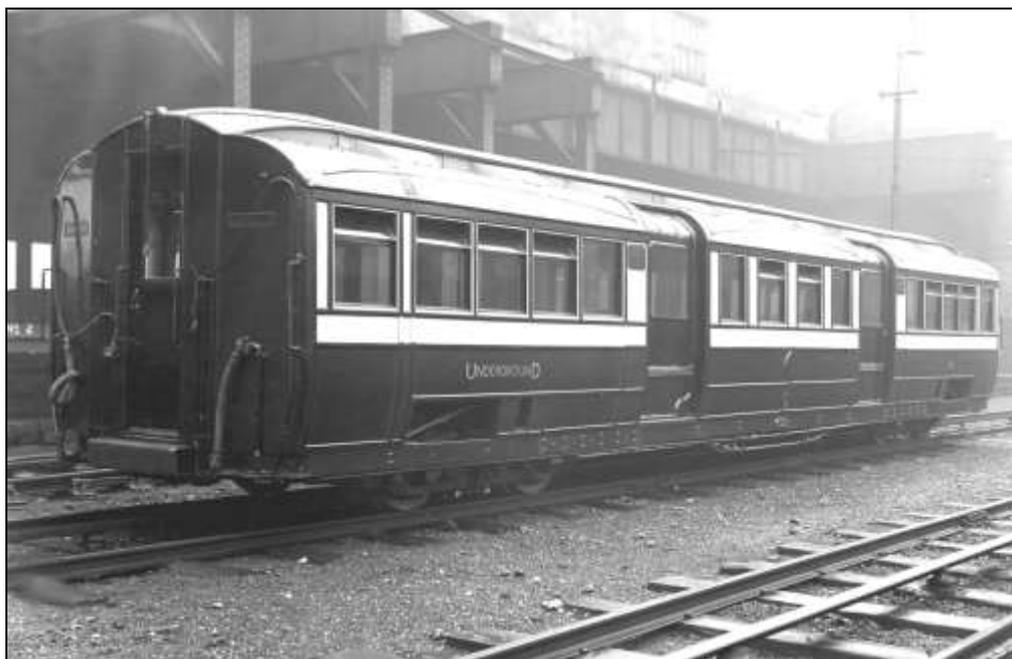
*Figure 4: CLR trailer car No. 40 standing outside the old loco shed at Wood Lane depot in January 1926 after its conversion to air door equipment. Two single leaf doors are provided on each side and the open platforms enclosed. The end coupling arrangements have been altered to suit. Photo: LT Museum.*
