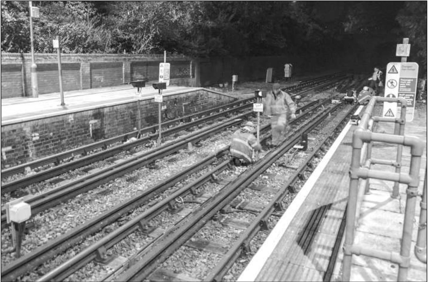
**Above:** For the train to reach the Ongar branch the fixed red lights in platform 1 at Epping had to be lowered for the train to pass over, the right-hand lamp already having been dealt with and pointwork in the process of being secured.
