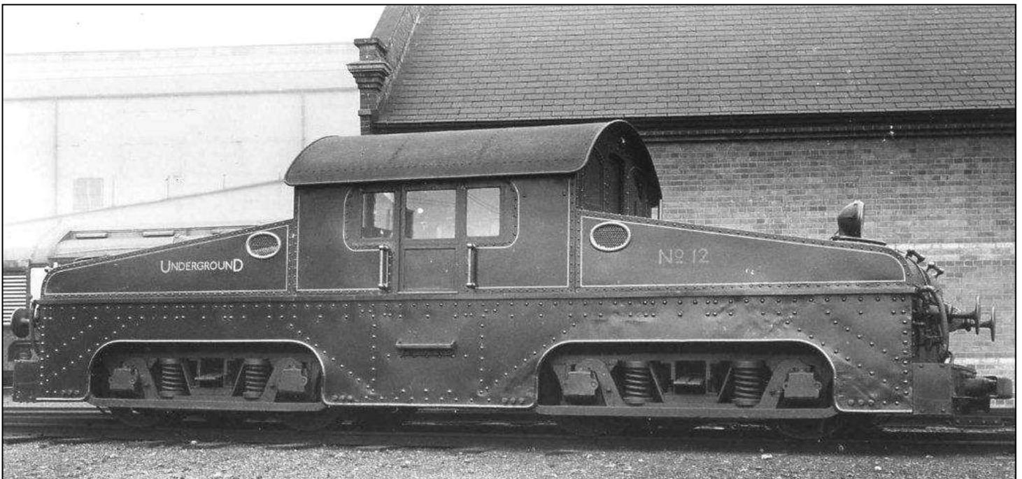
There were several photos of the CLR electric locomotives in their original condition in my articles but I did not include one of the remaining locomotives used for shunting. So here it is. This is the last surviving example, No.12, standing on the loop track next to the car shed in Wood Lane depot. The date is probably late-1920s. In the background, the halls built for the 1908 Franco-British exhibition can be seen. The present Westfield shopping centre was built on this site.
