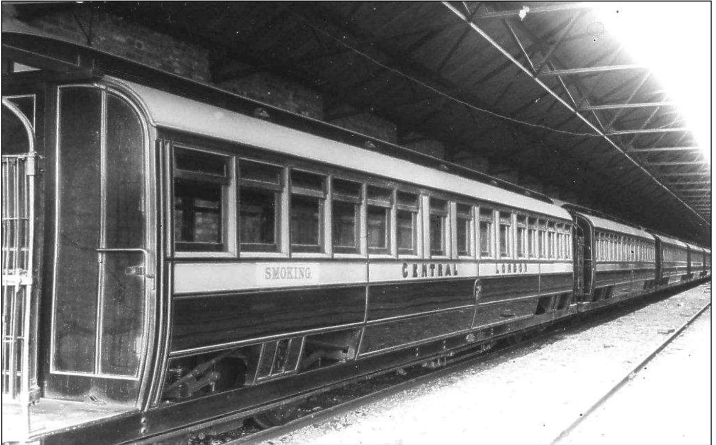
This photo shows a set of brand new trailer cars inside the shed at Wood Lane depot. Note the lack of car numbers. The car nearest the camera has SMOKING labels attached to the car sides where the car numbers were later displayed. The smoking signs then had to be moved to the saloon windows. This and other photos suggest that the smoking cars were located at the ends of each 7-car train.
