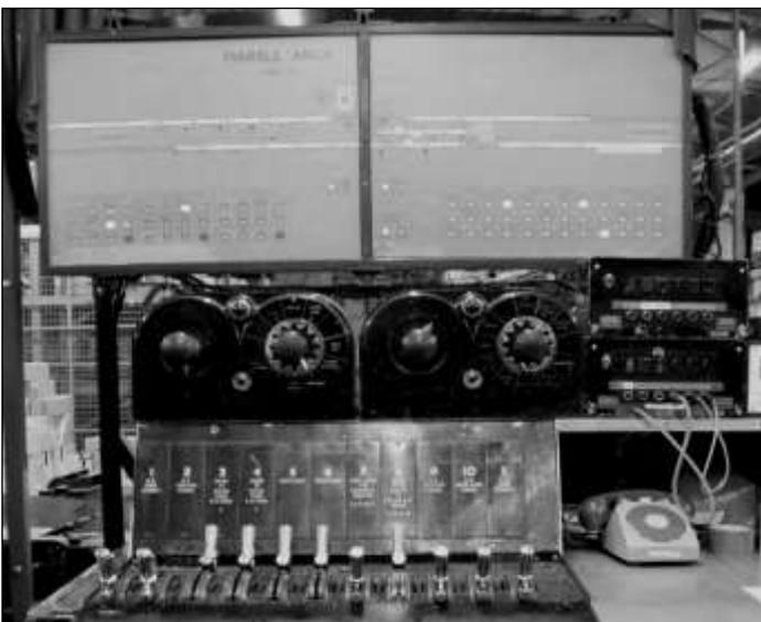
**Left:** The signal diagram for Marble Arch, underneath which is the train description apparatus. At the bottom is the 11-lever frame.
