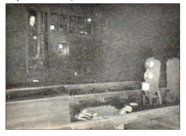
The signalbox (*Left*) was scooped out of the eastern tunnel wall and was accessed from an anonymous door set in the wall of the cab rank on the west side of St. Pancras station. The door led to a spiral staircase at the bottom of which another door led into the tunnel itself. To gain access to the box the tracks had to be crossed. (*Apologies for the poor photo – Ed.*).
