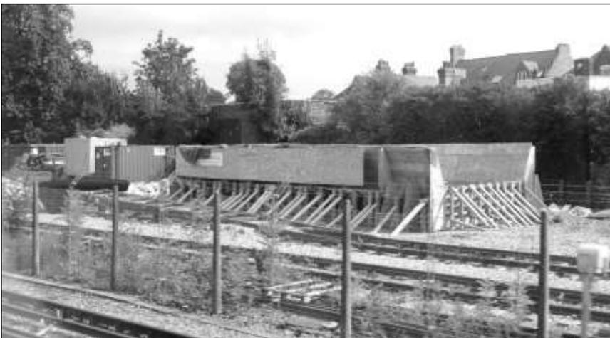
**NF 126/15** – Work on a world-first tunnelling project is underway that will significantly reduce the amount of repair work needed on the Metropolitan Line and disruption to passengers. The three-year project has involved the creation of a 15-metre replica of the Baker Street to Finchley Road tunnel, which allows the team to test materials and working methods beforehand for complex track renewal, ahead of work starting in June 2015. The original plan for im-
