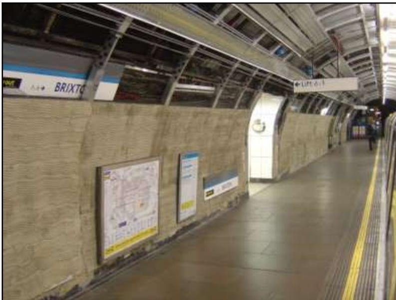
**BRIXTON** – There is nothing new to report regarding the escalator shaft and ticket hall. On the platforms the curved framework has been cemented for future new panelling (*left*) and now stands proud of the original tilework, marginally reducing the platform width.
