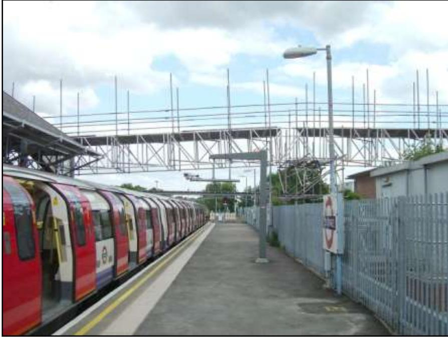
**EDGWARE** – Even though work has started here quite recently, there is much to see and report. A materials access 'bridge' has been erected across the south end of platform No.1 (*left*). All of the platforms 2/3 train shed has been scaffolded (*overleaf, top left and right*) to enable work to take place on the train shed roof. Temporary lighting has been installed and preliminary cabling work has begun. All three platforms have tactile strips.
