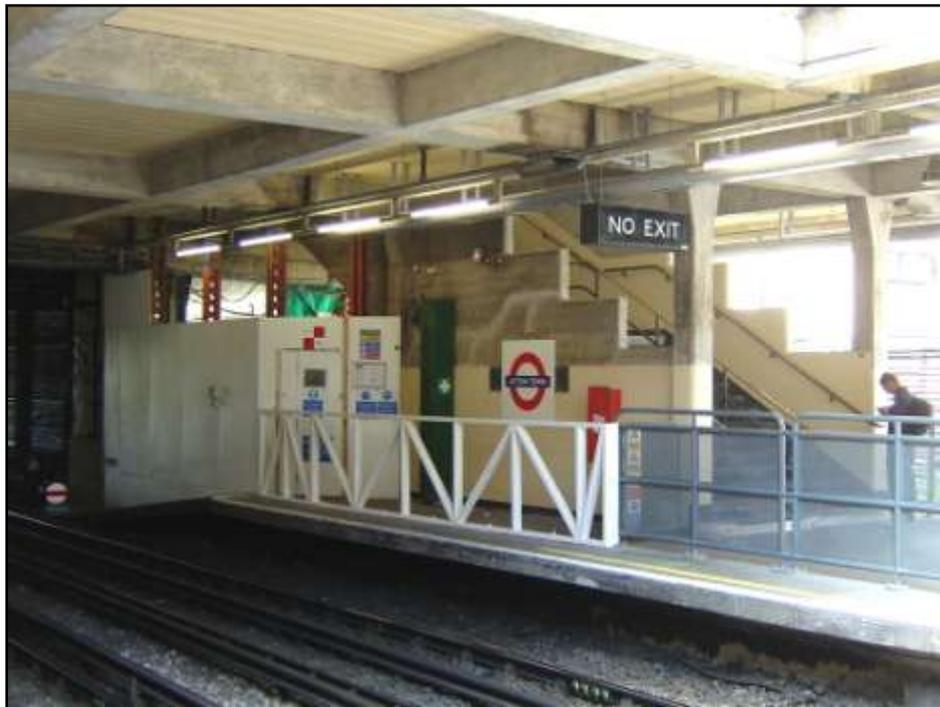
**Left:** The west end of the eastbound platform at Acton Town on 19 June 2008 showing the protection provided for the construction of the new MIP lift.
