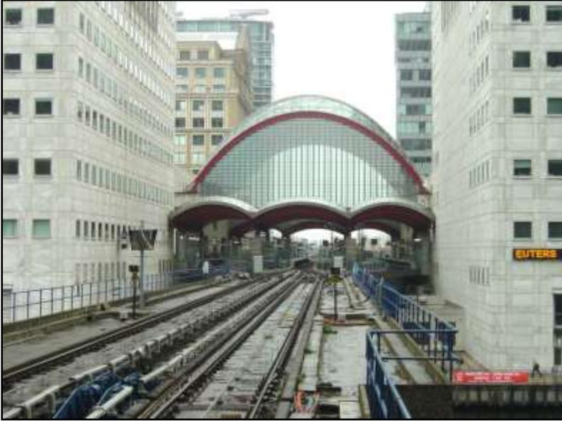
The replacement station at Heron Quays was built to accommodate three-vehicle trains and will therefore not need lengthening. This view (*left*) looks north from the north end of the southbound platform to Canary Wharf. The only clue as to where the original Heron Quays station used to be is with the OPO mirror that remains in splendid isolation north of the new station on the centre left of the photograph. The old station was thus even closer to Canary Wharf station!
