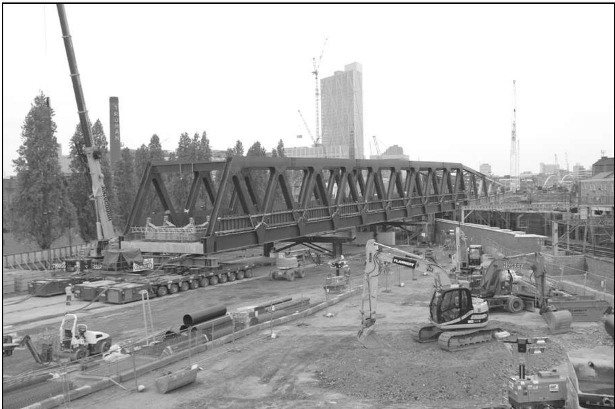
**Previous Page:** (Lower) Major bridge works have been a feature of the East London Line re-construction and extension earlier this year. Following on from the positioning of the bowstring bridge over Shoreditch High Street on 29 March (*lower back cover, this issue*), the girder bridge to carry the ELL over the Liverpool Street
