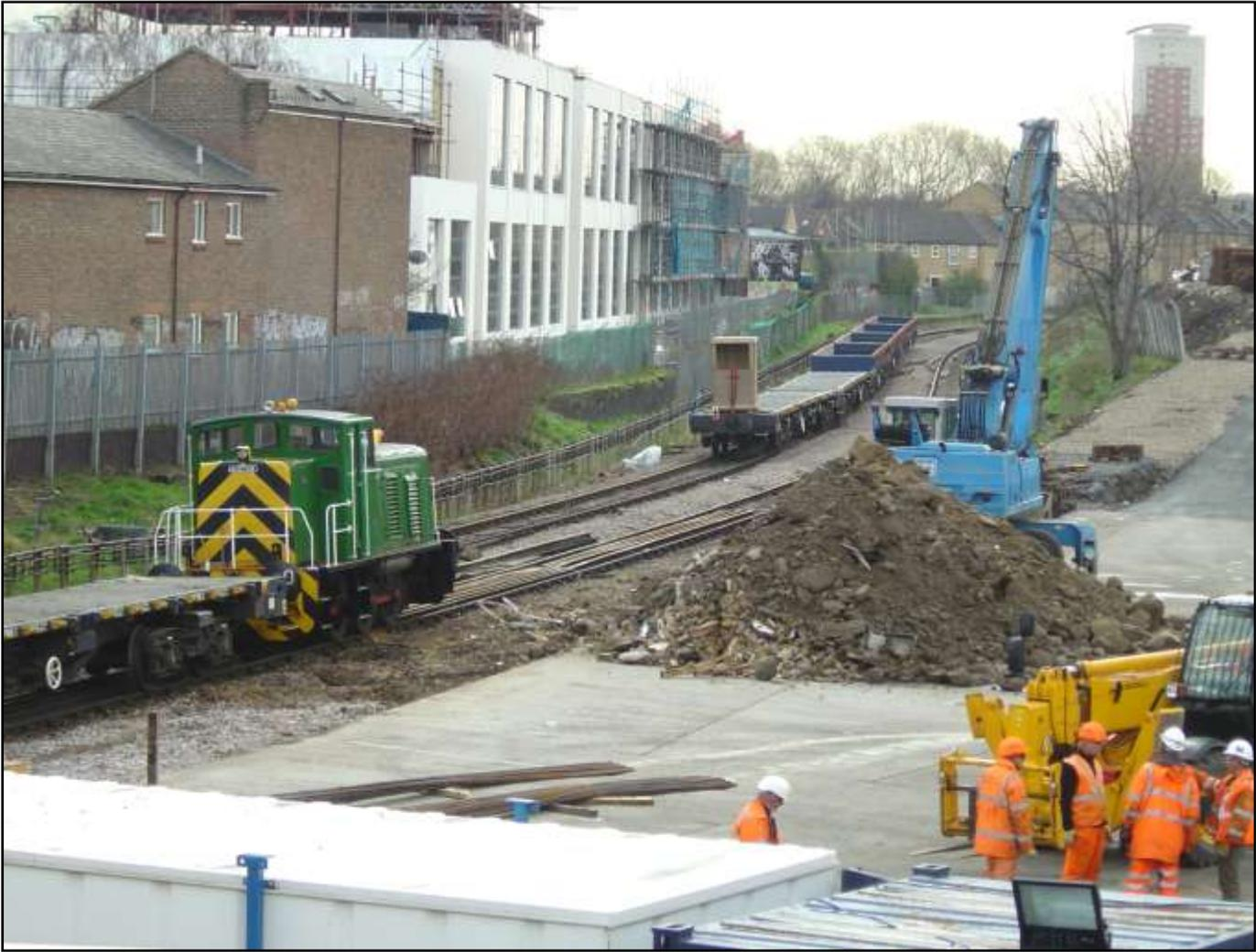
**Above:** Looking south-east from Trundleys Road footbridge on 27 March 2008, one of the Ruston diesel locomotives is seen on the left of the photograph on the northbound East London Line while various wagons, without a locomotive, are seen on the southbound. Much of the conductor rail in this area has been removed. The structure on the flat wagon is a rudimentary “guard’s van” incorporating a brake setter and air horn (to assist propelling movements).
