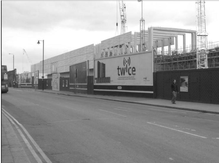
**Left:** Construction of the East London Line extension proceeds. On 16 September 2008 the superstructure of Shoreditch High Street station was well in evidence alongside Bethnal Green Road. The concrete boxing in of the line is being taken as far as the bow-string bridge over Shoreditch High Street to acoustically isolate the line from future building developments.
