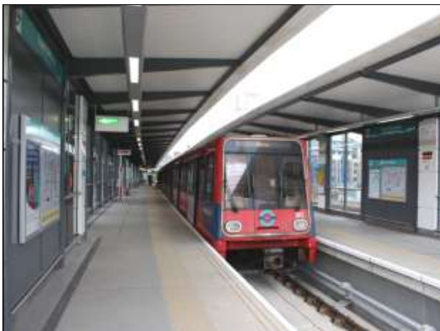
The rebuilt Tower Gateway station as seen on 27 March 2009, with the single track terminus and platforms either side clearly visible.
