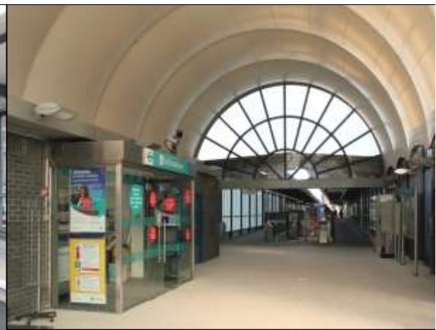
The refurbished ticket hall of Tower Gateway on reopening day. The roof appears to be covered in a canvas type material.
