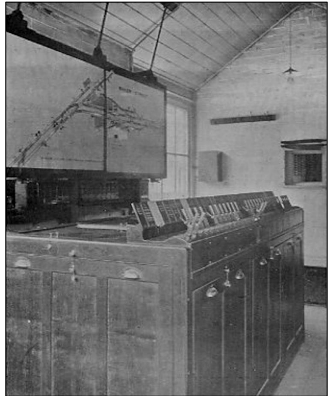
Figure 4 (Left): Westinghouse Style M1 frame in Aldgate signal box used from 1909-1927. This box was located at the end of the Circle Line Inner Rail platform. As part of the station rebuilding in 1927, a new box was built further west and this frame was moved there. It was replaced when a new box was built over the station and opened in 1946. The M1 frame design is quite distinct compared with the Style B frame. It looks as if the levers were added as an afterthought. Note how the lever nameplates are stand alone rather than being incorporated into the cabinet as on the Style B frame. Photo: Originally Westinghouse.
