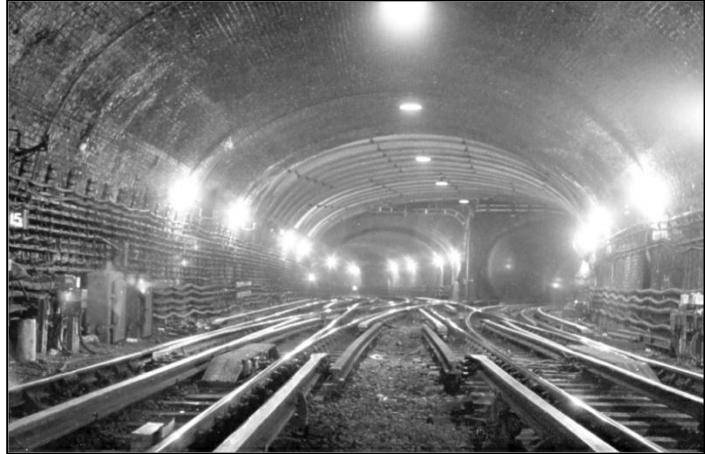
*Left: Praed Street Junction looking west, with the lines to Paddington (Circle) to the left and to Paddington (H&C) to the right. Note the iron structure at the top of the tunnel just above the centre. This also appears clearly in an original print (Below, Left) around the time of opening with broad gauge steam traction, but looking in the opposite direction.*
