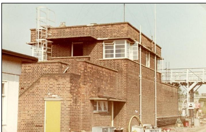
Located at the south end of the depot between the 'Klondyke' tracks and main depot, this opened on 27 June 1938, comprising an N style frame with 83 levers. It closed on 29 October 1988 with control to Baker Street signalling control centre.
