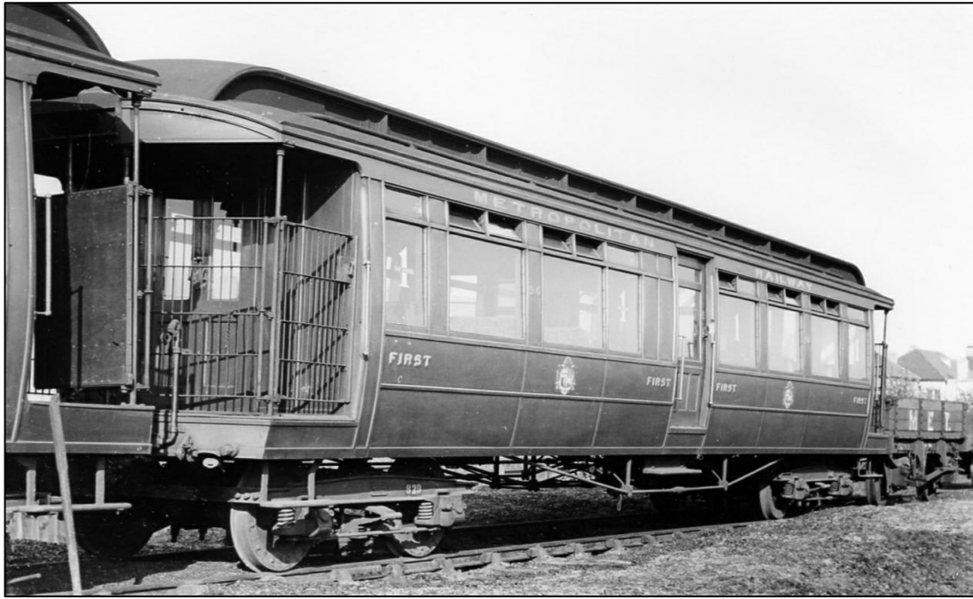
Figure 4: The wooden bodied 1st class GN&C trailer car No.94 awaiting scrapping at Neasden. The car is in Metropolitan Railway livery and hasn't been renumbered into the LPTB series. The side window adjacent to the centre doorway has been blanked off as part of the conversion to first class. Note the adjacent car platform has plain steel sheeting over the gate. A number of cars had this feature. Photo: B.R. Hardy collection.
