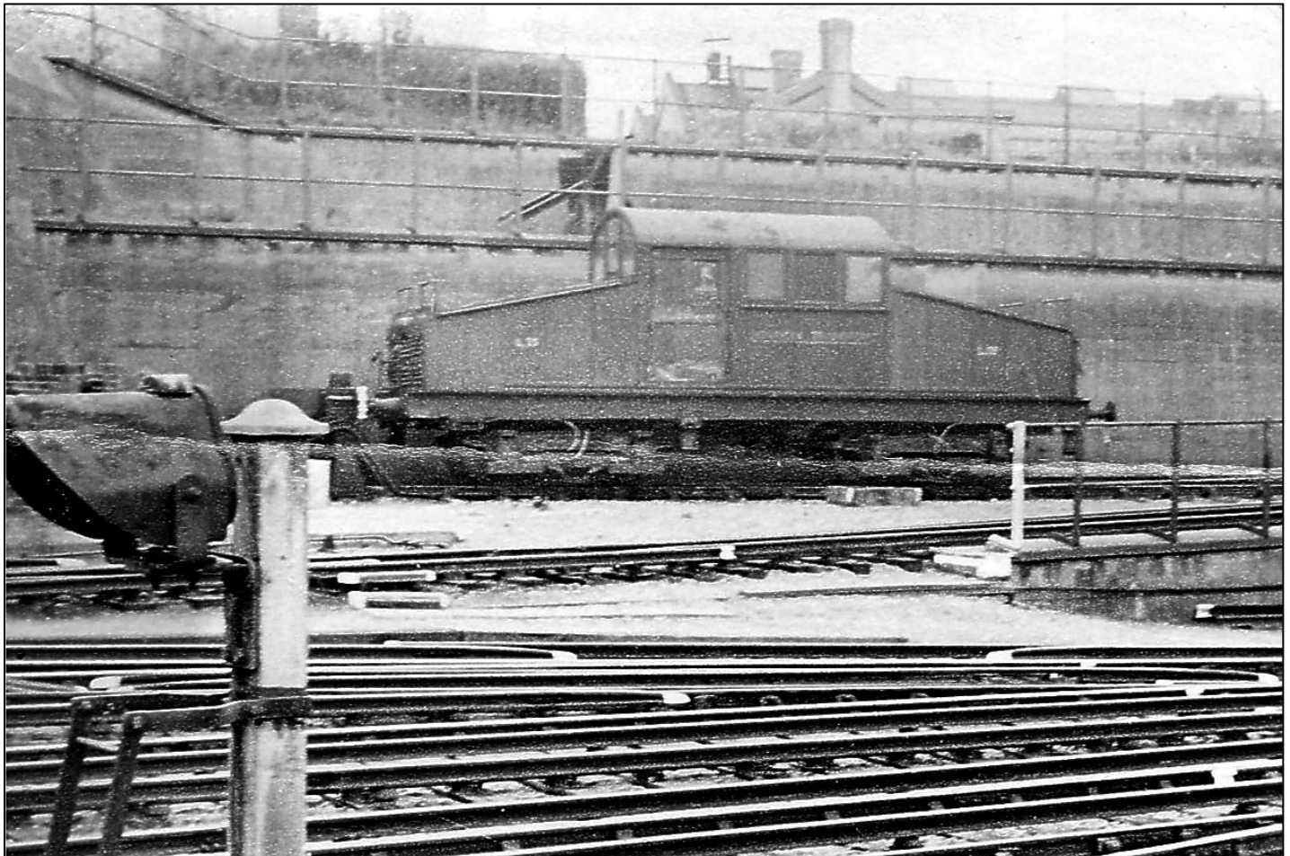
Figure 7: The former Metropolitan Railway electric locomotive in the yard at Drayton Park displaying the title London Transport and the number L33. The photo was taken after May 1939 as the loco has its shoe gear modified for standard Underground 4-rail current collection. The yard also has been relaid with the standard 4-rail system. It is difficult to see but there is no evidence of tube stock couplings to allow it to shunt tube stock. Photo: B.R. Hardy collection.
