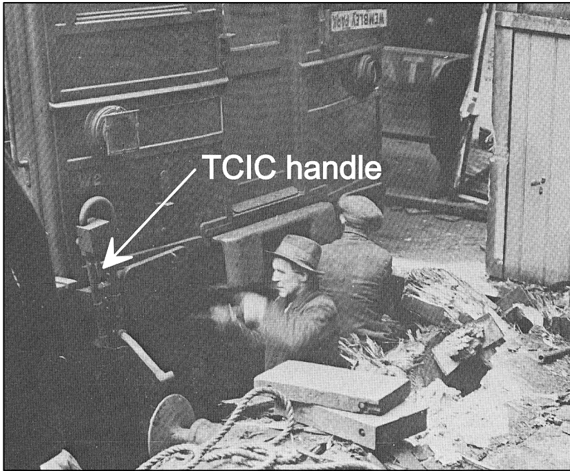
Figure 7: This photo of a train being rescued after a buffer stop collision at Moorgate shows the pipework on the front of the train for the tripcock isolating cock. The cock handle can be seen at the bottom of the switchbox. This modification was introduced sometime around 1914-1916 on the Metropolitan's electric stock. Photo: Collection B.R. Hardy.
