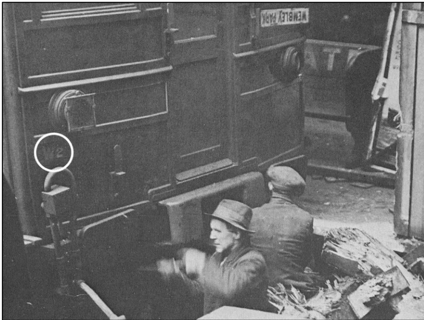
Figure 3: The breakdown gang hard at work after a buffer stop collision at Moorgate in the early 1920s. The interest for us here is that close examination of the car end shows the code W2 (circled). The W indicates a BW equipped train. Probably the '2' indicates a 200hp motor car as this was 1913 Stock. Photo: Author's collection.
