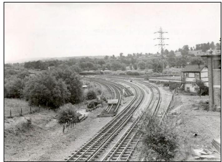
**Above:** In June 1950, the track at Watford South Junction was slewed on a new alignment 30ft west of the present from 1,000ft north of Watford South Junction to 1,500ft south of Watford South Junction, to allow bridges MR78, MR80 and MR81 to be taken out of use. Watford Road Junction signal box may be seen in both photos, along with Croxleyhall substation in the left hand photo.
