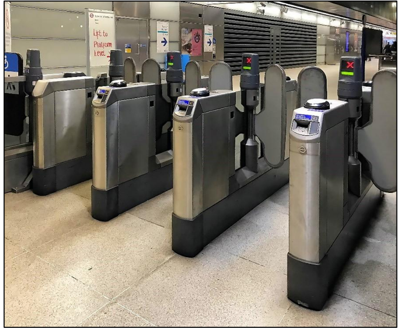
First-generation electric E1 gates at Canary Wharf. These are all bidirectional and can be set for either 'entry' or 'exit' mode. Note the small LT roundel feature below the ticket entry slot, and the Contactless readers fitted retrospectively on top of the stanchions.
